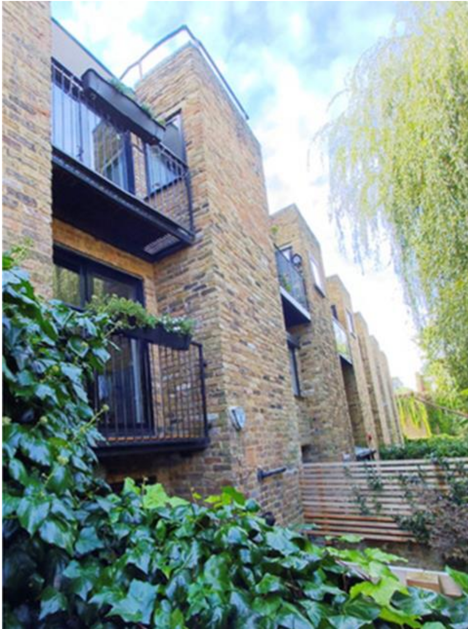
Rear elevation of terrace (Note: Existing windows added to rear bays at 2 nd floor level)
