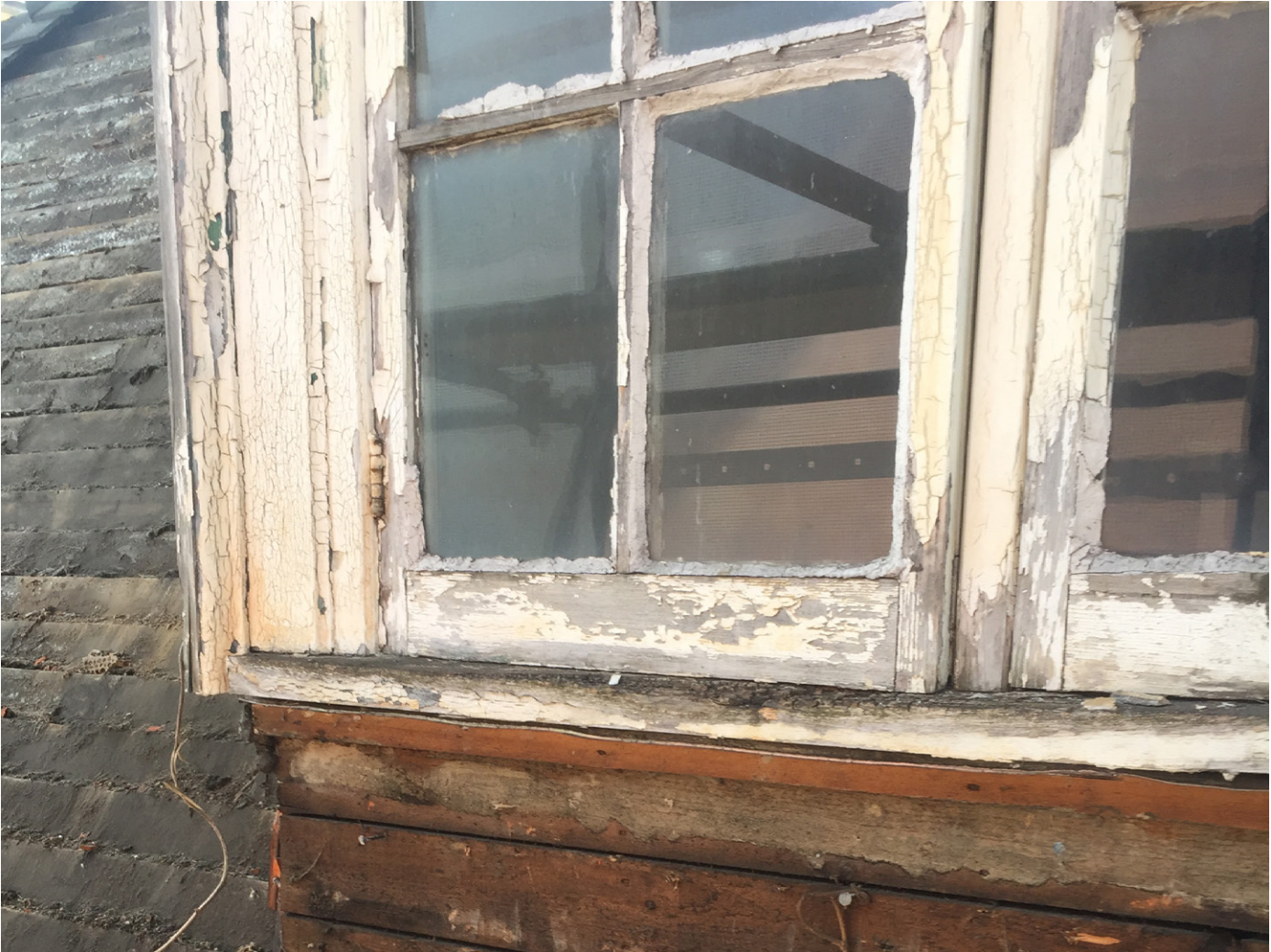
Existing timber casement window condition
