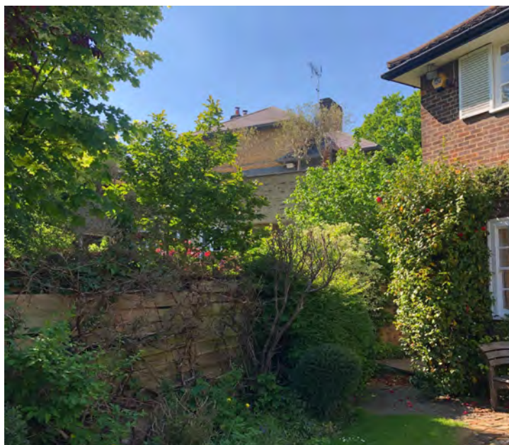
(Photo of the retaining wall, and boundary with the end of 18 Frognal Way's garden)
