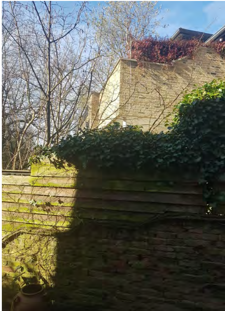
(Photos looking up at 18 Frogna1 Way, to show its greater elevation and taller stature)
