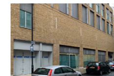
Current view along Betterton Street
