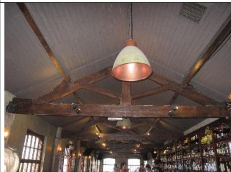
King post roof trusses at western range of West Yard second half of C19 largely altered in 1970s
