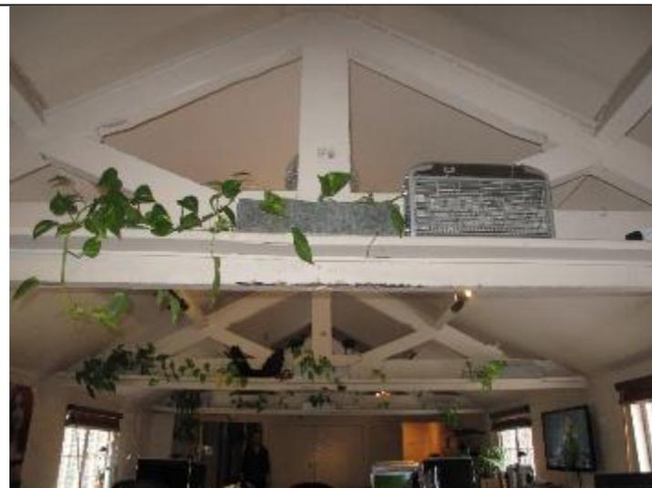
Northern range of West Yard, king post roof trusses, second half of C19, altered in 1970s
