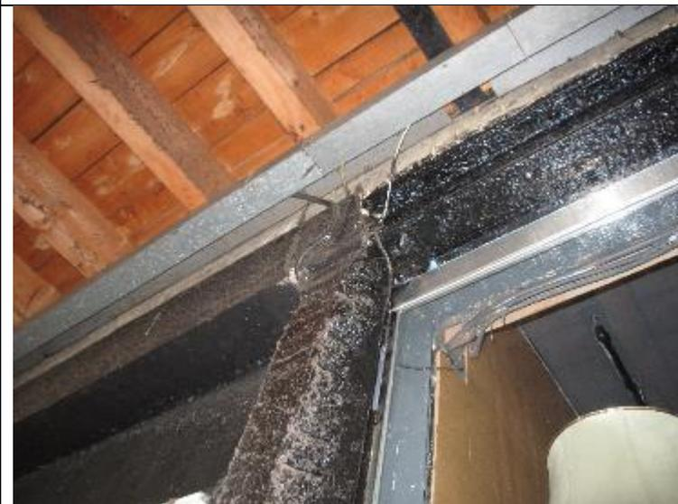
Metallic structure to the western range of West Yard, former transit-shed, second half of C19 cast in concrete probably in 1970s
