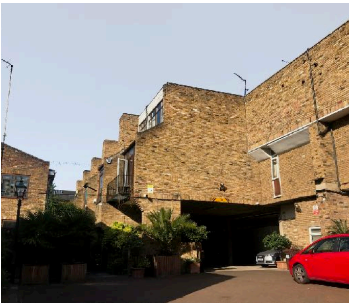
Existing houses with abrupt flat roof line
