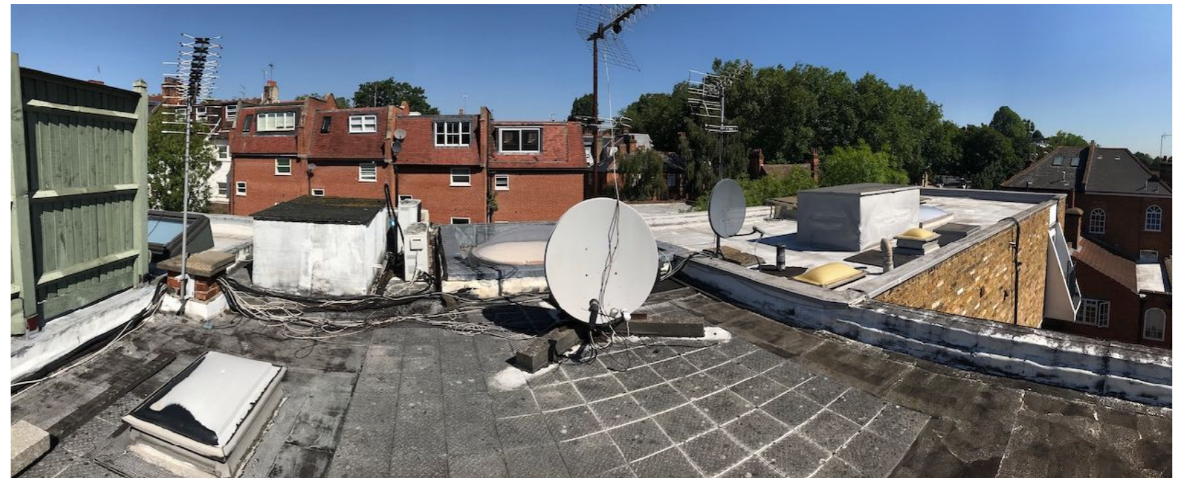
Roof of 23 Maryon Mews
