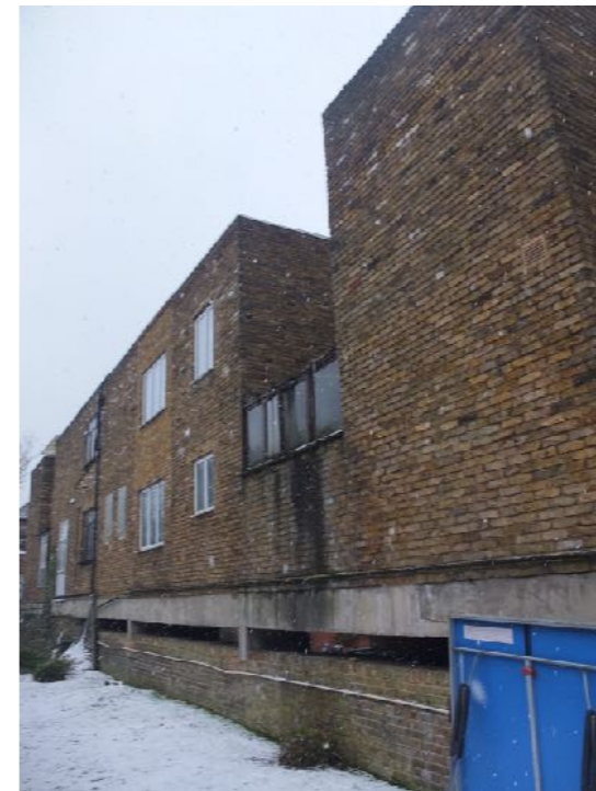
View north west
