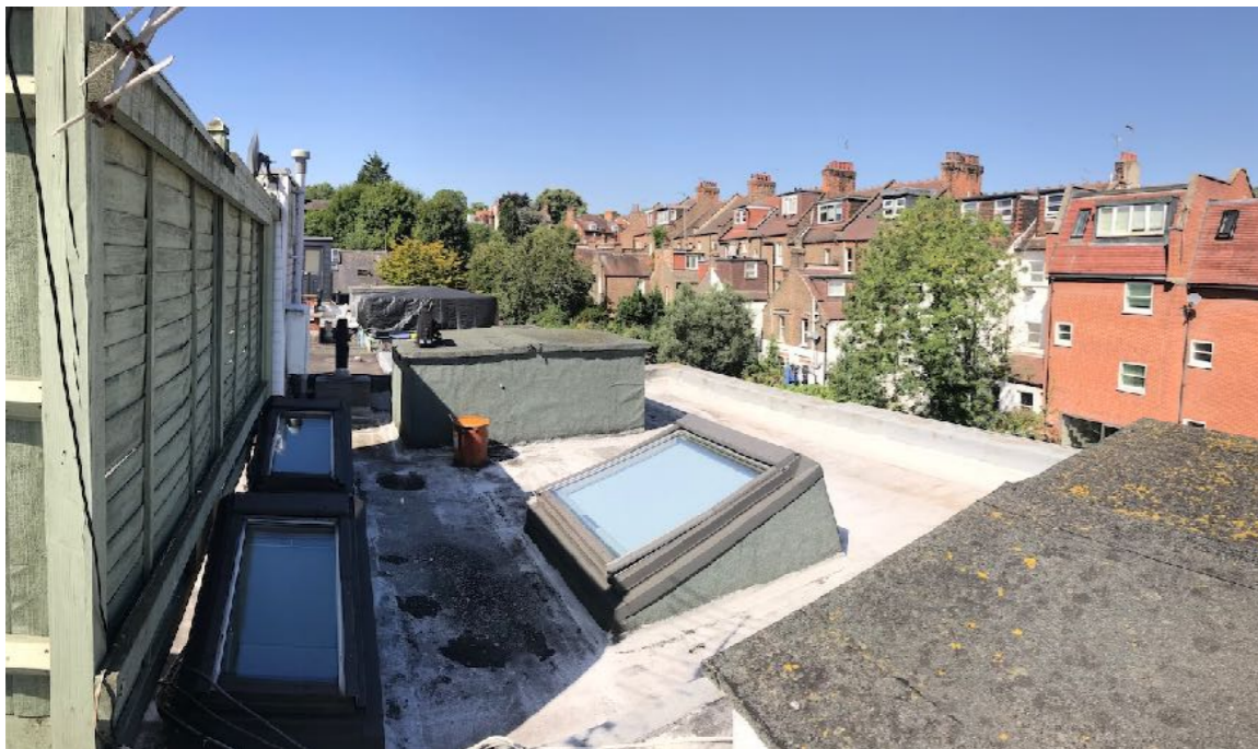
North side of Roof of 22 Maryon Mews
