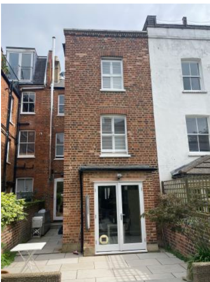
Fig 02: rear of 3 Mackeson Road : existing
