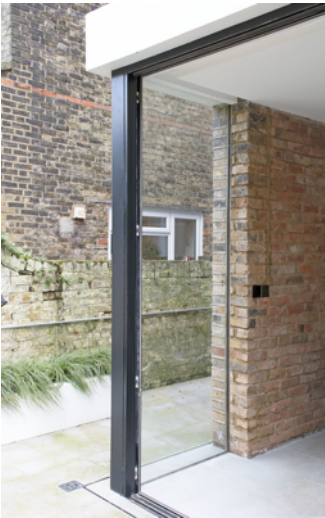
fixed and sliding corner glazing
