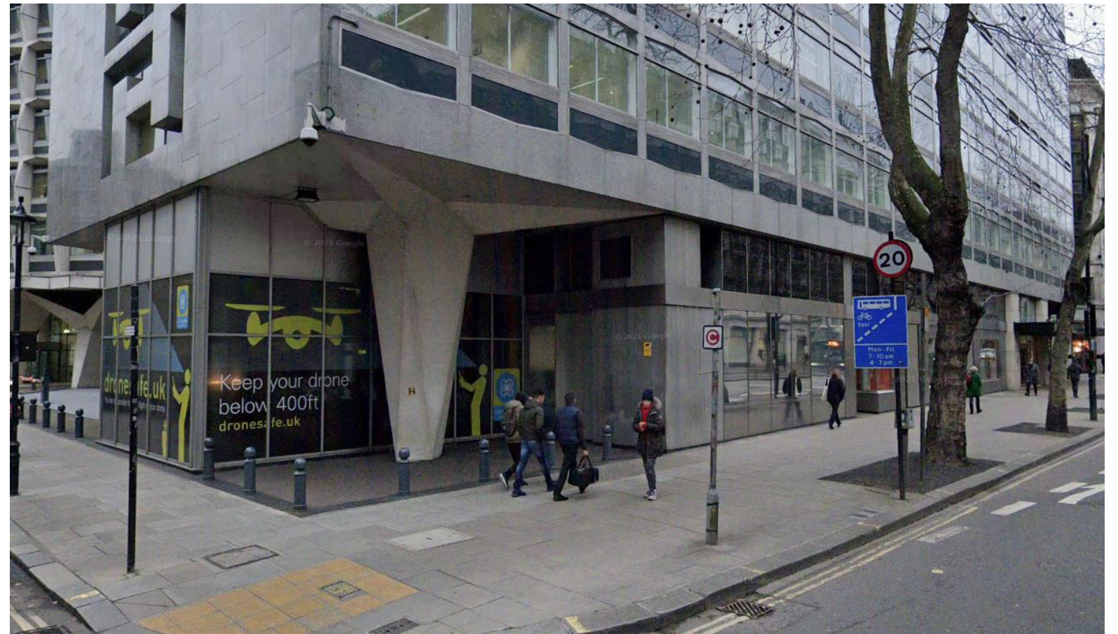
Fig. 2.0.12 Site photo - existing Kingsway reception
