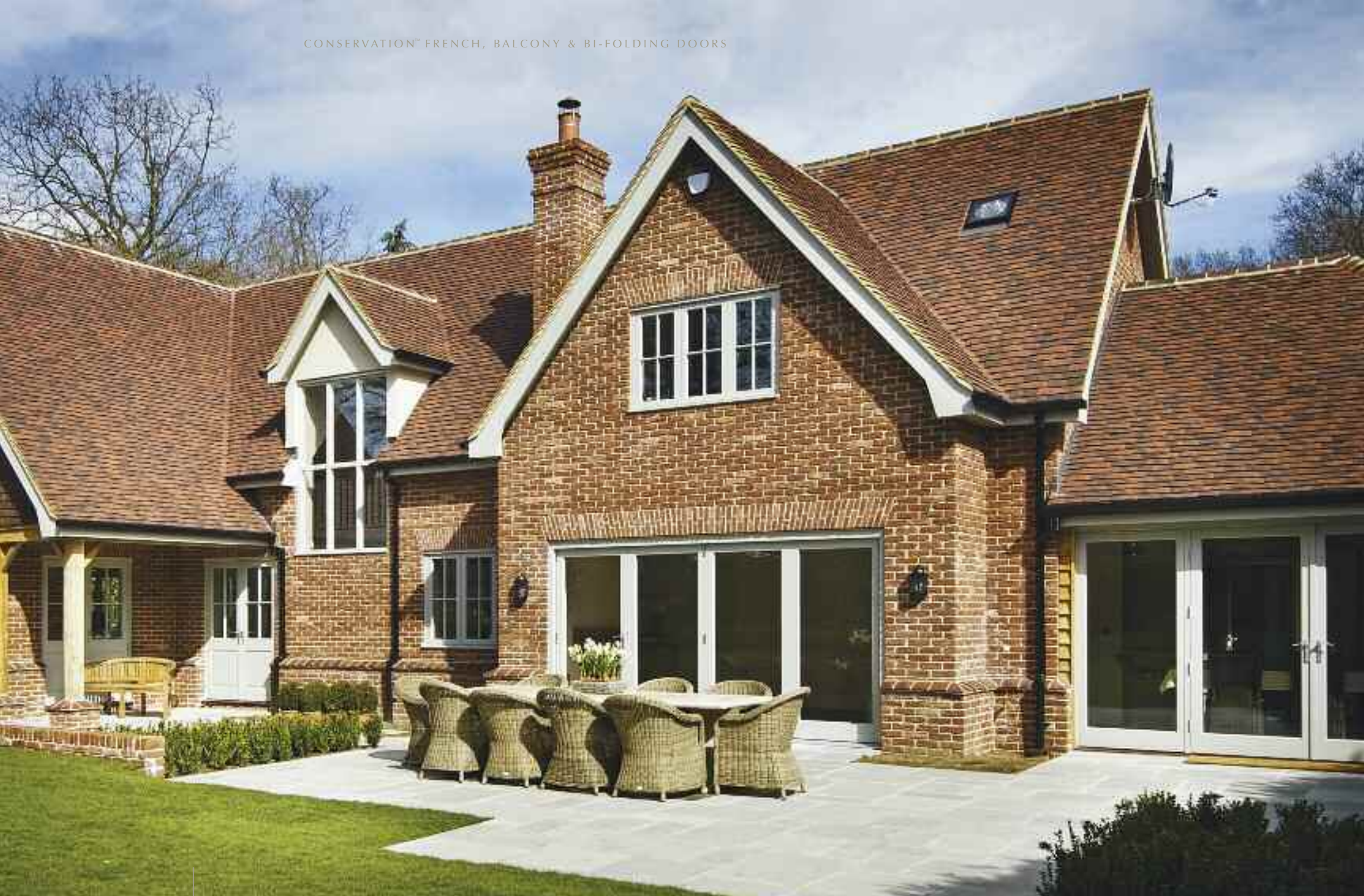
MAIN IMAGE DANBURY, ESSEX Conservation™ range products throughout this new build give a traditional feel, with Bi-Folding doors providing a true link to the garden.
