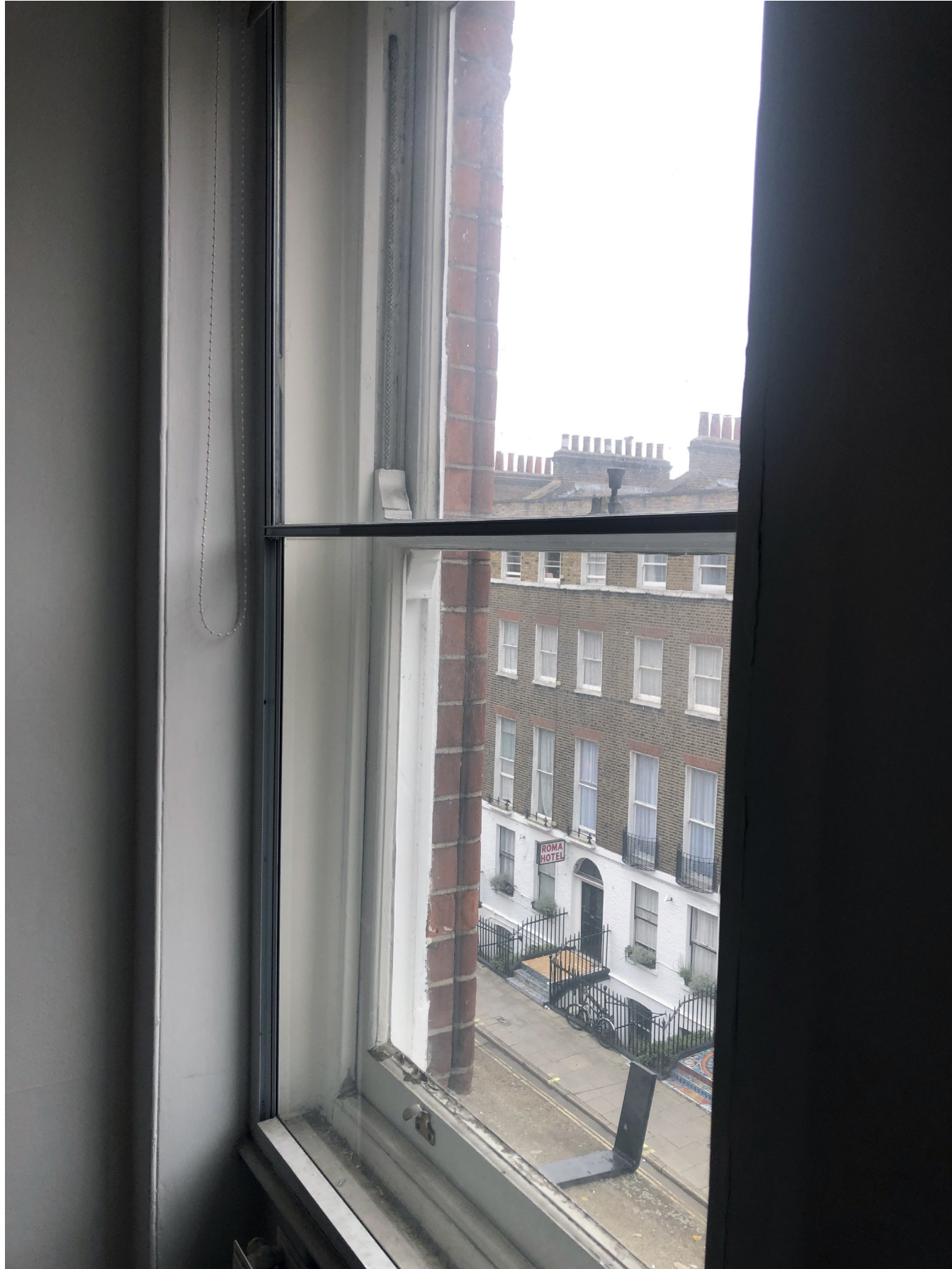
Internal, secondary glazing layer remains ineffective and obstructs maintenance
