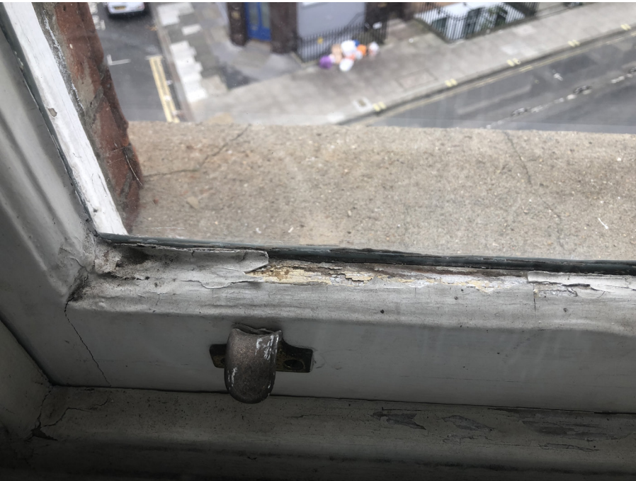
Timber starting to rot and peel away, dilapidated throughout
