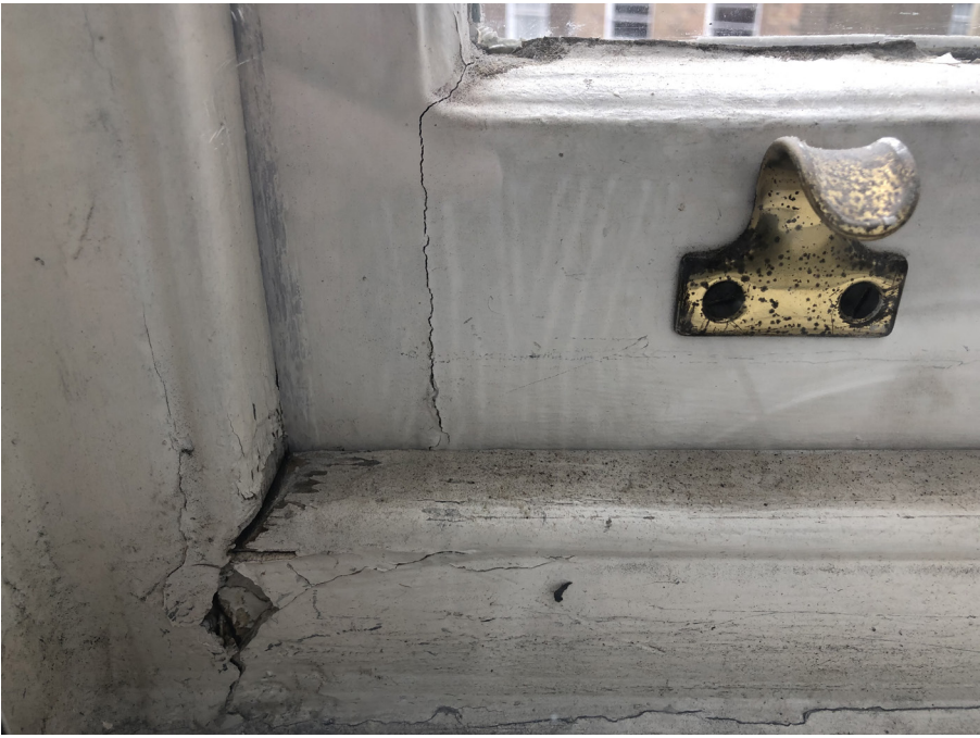
Structural issues from rotting
