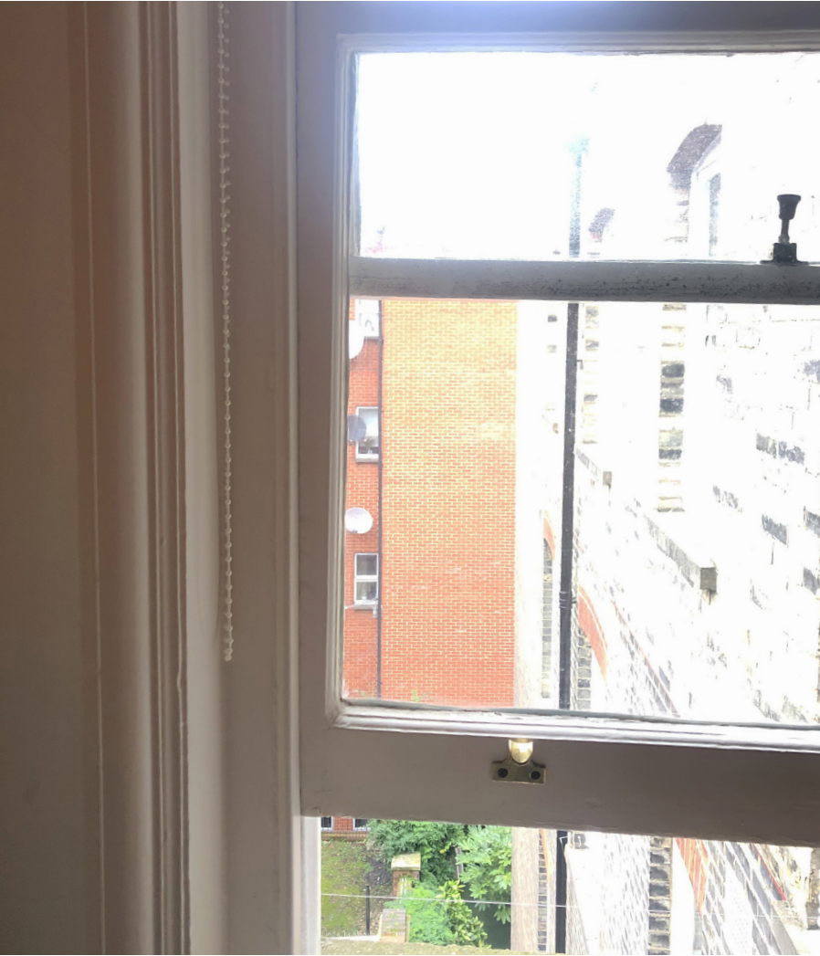
Sliding system no longer operating smoothly due to warping
