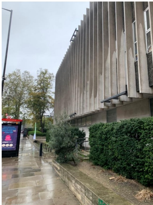
Figure 7 - General view_West elevation
