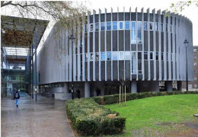
Figure 5 - General view_North elevation
