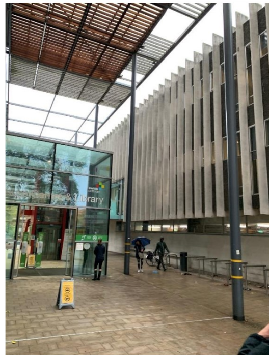
Figure 7 - General view_East elevation
