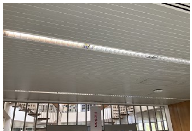
General view of perforated metal suspended ceiling with integrated lighting
