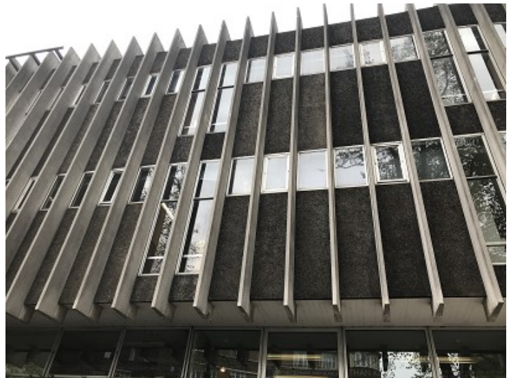
Detail view showing Spence's arrangement of windows corresponding with adjacent vertical and horizontal elements
