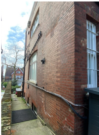
STITCHED BRICKWORK OF HISTORIC DOOR OPENING ON SIDE ELEVATION
