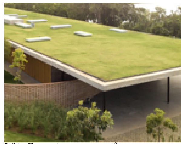
LS1: Extensive green roof
