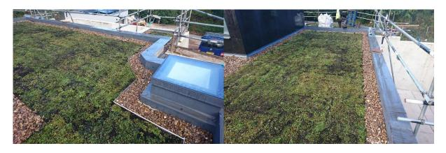
Considerations: Green roof systems include living products which must be installed on day of delivery and watered immediately upon installation. If watering is not implemented immediately and for the first 12 weeks in situ, Sky Garden Ltd cannot take responsibility for the growth and success of the vegetation. This is especially important during the Spring and Autumn period each year. For pitched roofs over 7.5 degrees, we would recommend an irrigation system to be installed with the roof.
