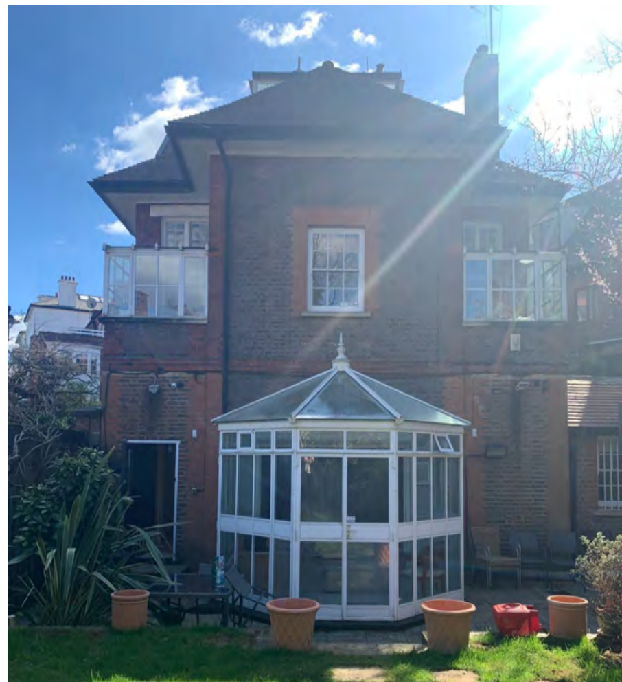
Figure 6: Studio House the rear of the principal listed building
