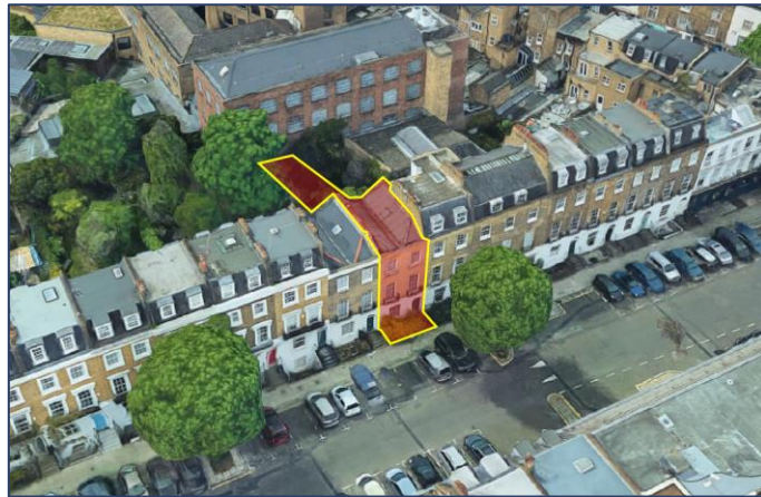
Figure 1- Aerial view of the site from the West
