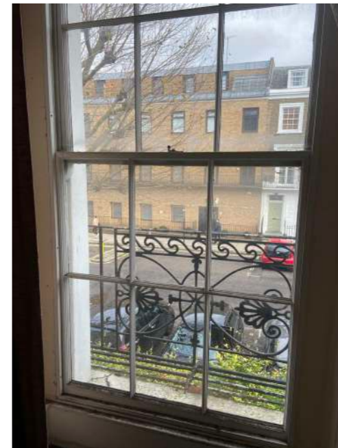
Front Room - showing replacement windows and external balconies
