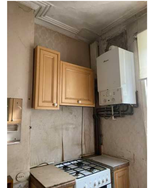
Rear Reception Room - significant damage to existing cornice, pipework and boiler/flue outlets
