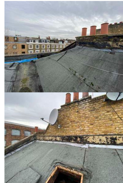
Existing Felt Roof
