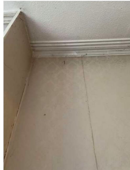
Front Reception Room - cornice and existing in-built joinery cutting through cornice
