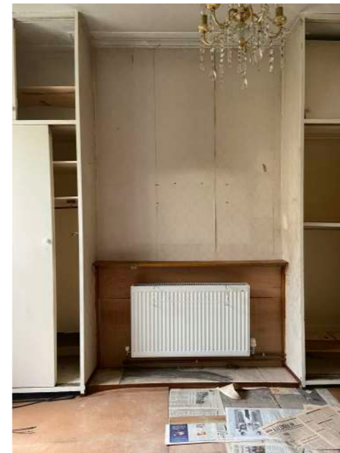
Front Reception Room - showing in-built joinery, chimney breasts present to all main rooms, no fireplaces present
