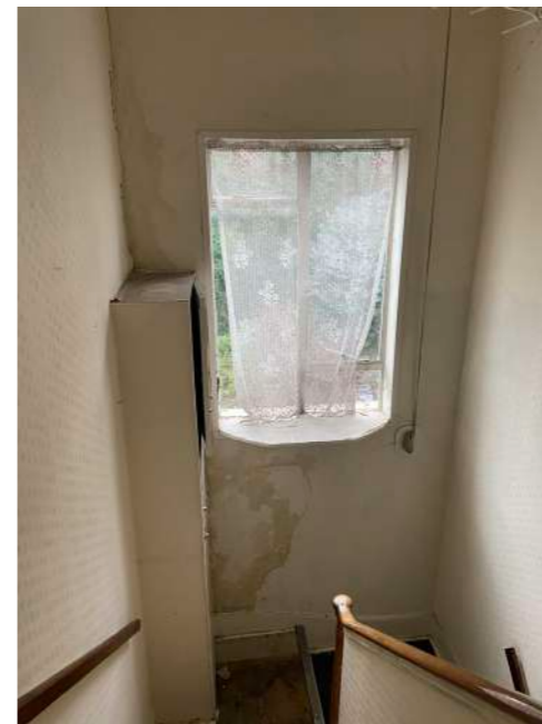
Stairs - looking down to 20th Century metal window and cupboard
