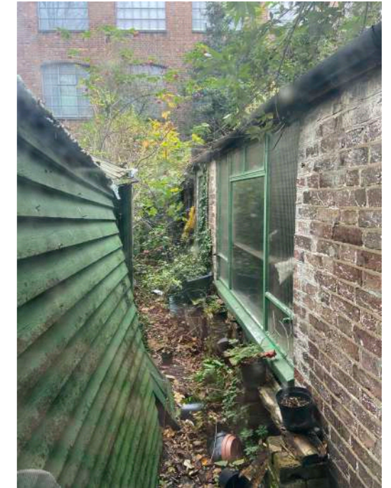
Existing C20 Outrigger and Timber Outbuilding
