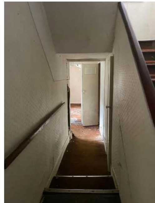
Hallway/Stairs - Original stairs with boarding to handrails, to be returned to original detail
