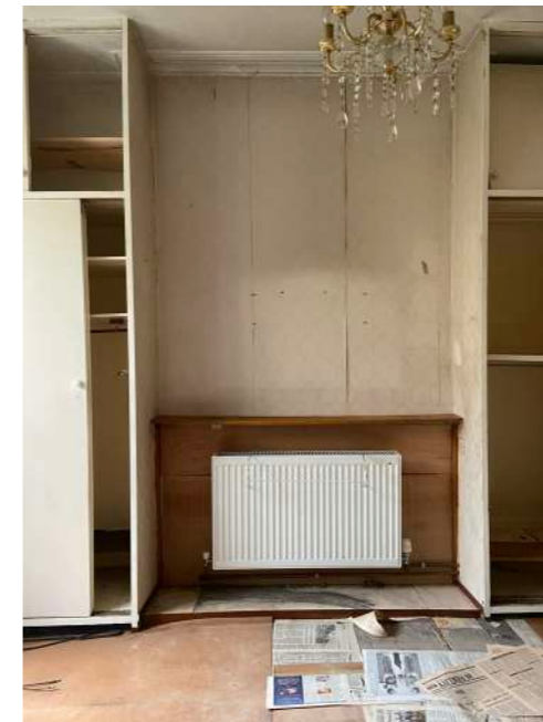
Front Reception Room - showing in-built joinery, chimney breasts present to all main rooms, no fireplaces present
