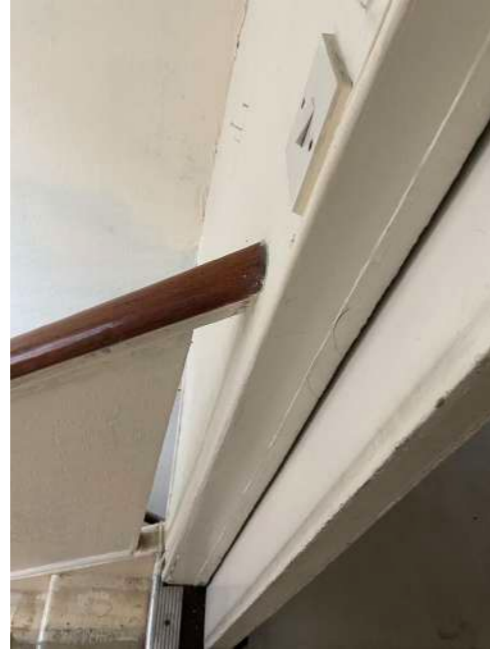
Stairs/Landing - looking up to Second Floor, original handrail removed to allow for partition
