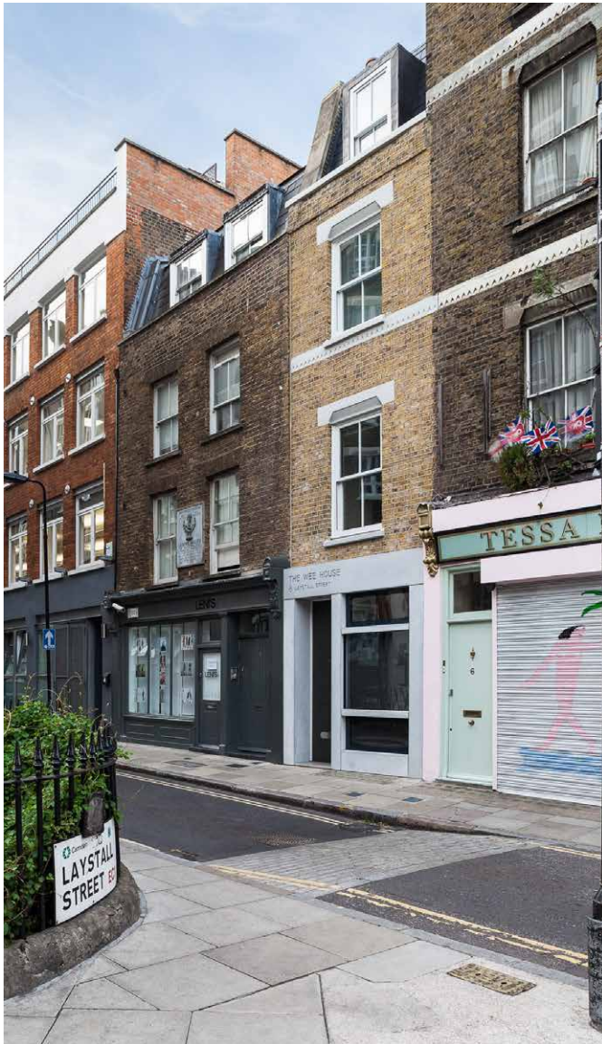
Views of the street frontage as existing
