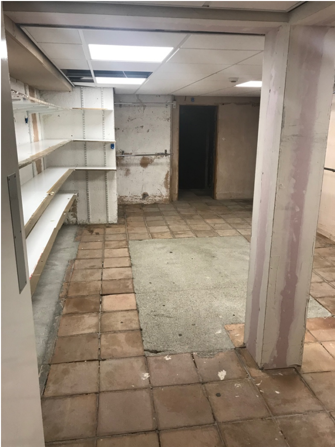
13: Existing Basement Stock Room
