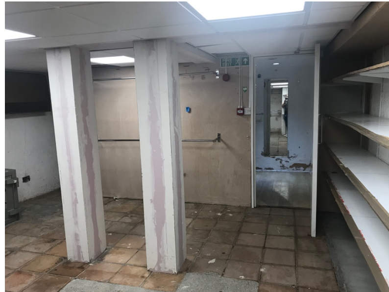
12: Existing Basement Stock Room
