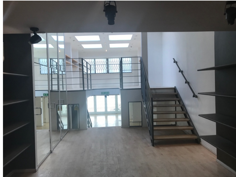
02: Existing Ground Floor Rear Sales Area
