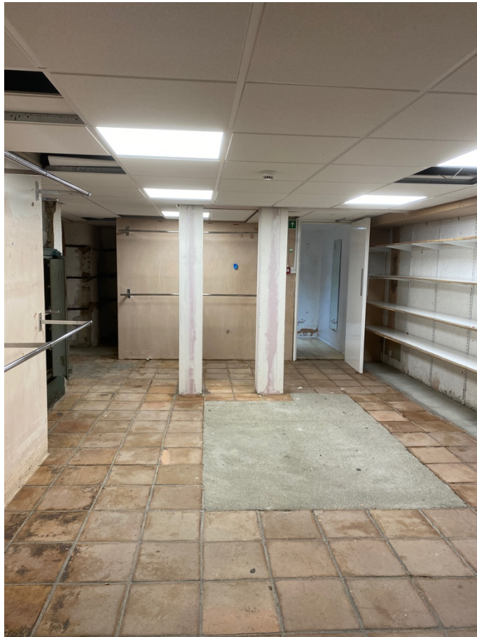
14: Existing Basement Stock Room
