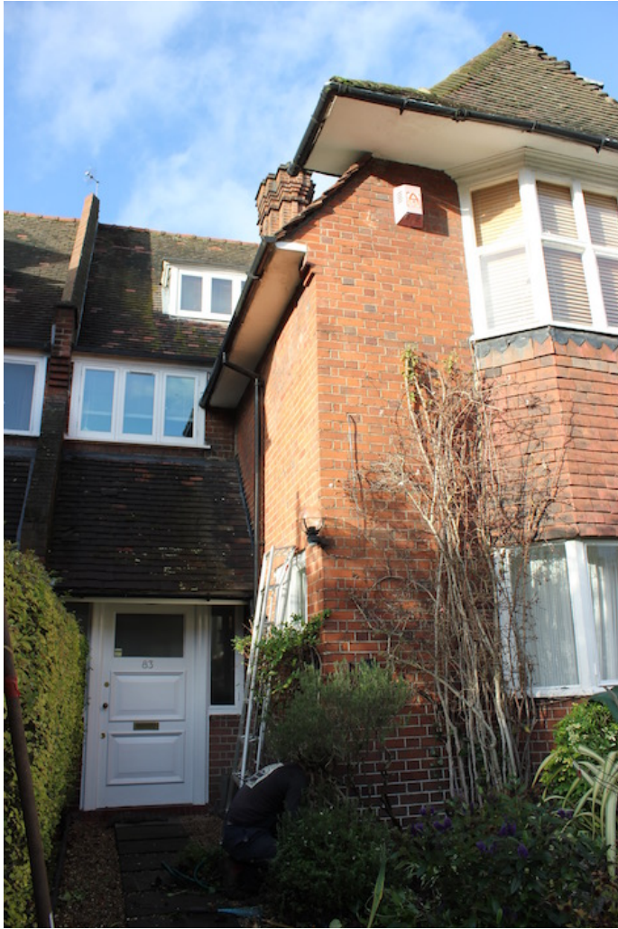
FIGURE 2: VIEW OF FRONT OF HOUSE, INCLUDING MAIN ENTRANCE
