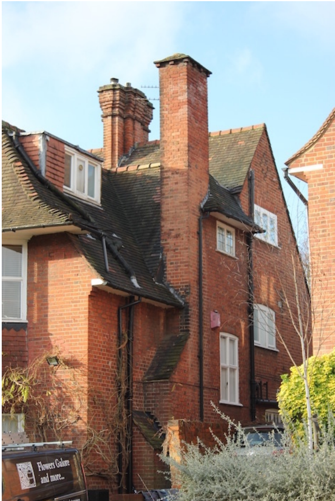
FIGURE 1: VIEW OF SIDE ELEVATION AND ROOFSCAPE
