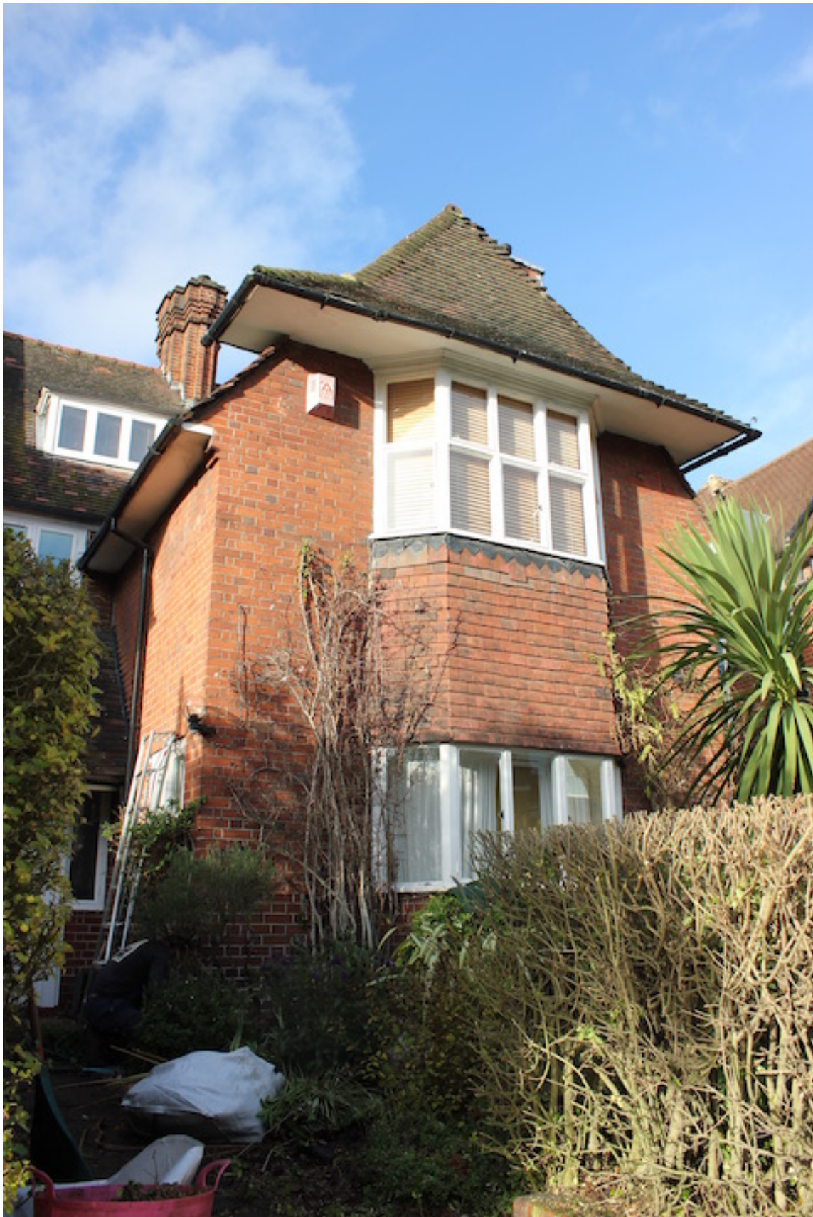
FIGURE 4: VIEW OF FRONT OF HOUSE FROM STREET
