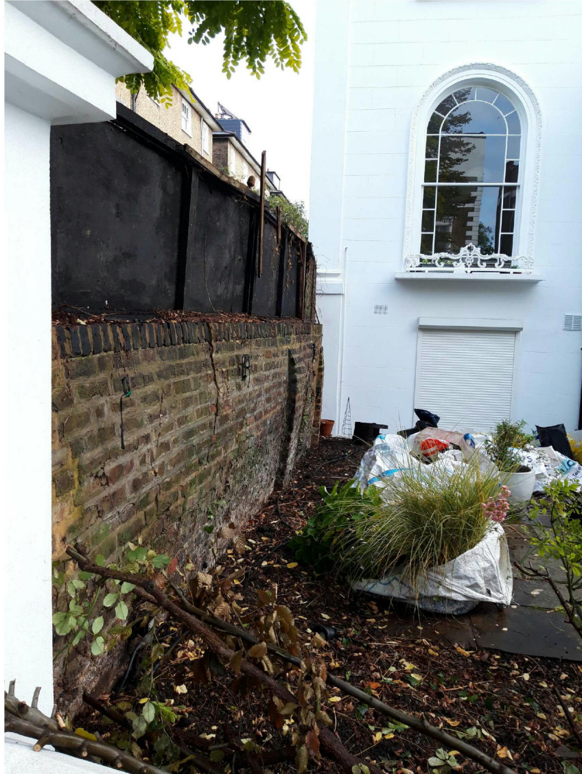
General view along wall
