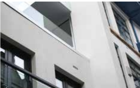
Existing white render, and frameless glazed balustrade
