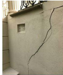
Left side of Portico and steps evidence of low level crack
