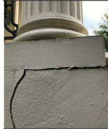
Crack widens to 5 mm as it reaches Portico
