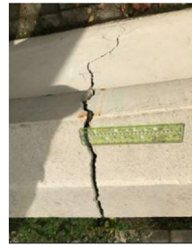
8mm full height wall crack extending through capping
