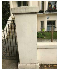
Pillar at front leaning to the left and towards pavement, gate will not close
