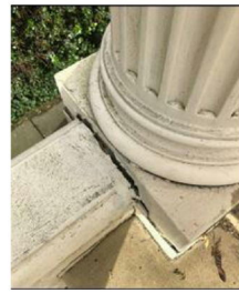
Portico Column separating slightly from stairwell
