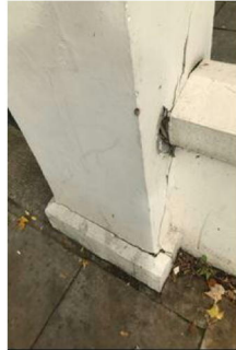
Gate pillar - wall movement around joint
