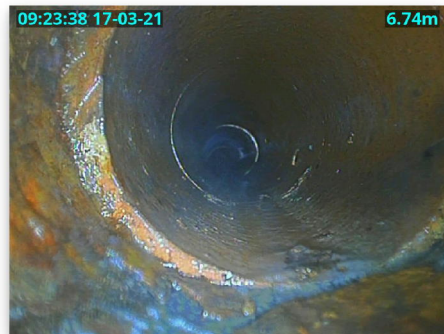
Fig 1.4: Line 1, cracking
