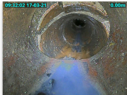
Fig 1.2: Line 4, displaced interceptor trap
