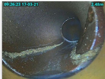
Fig 1.1: Line 2, joint displacement
