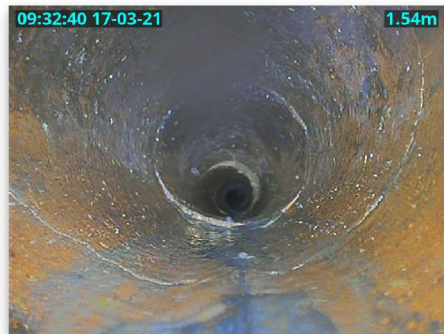
Fig 1.3: Line 4, cracking
