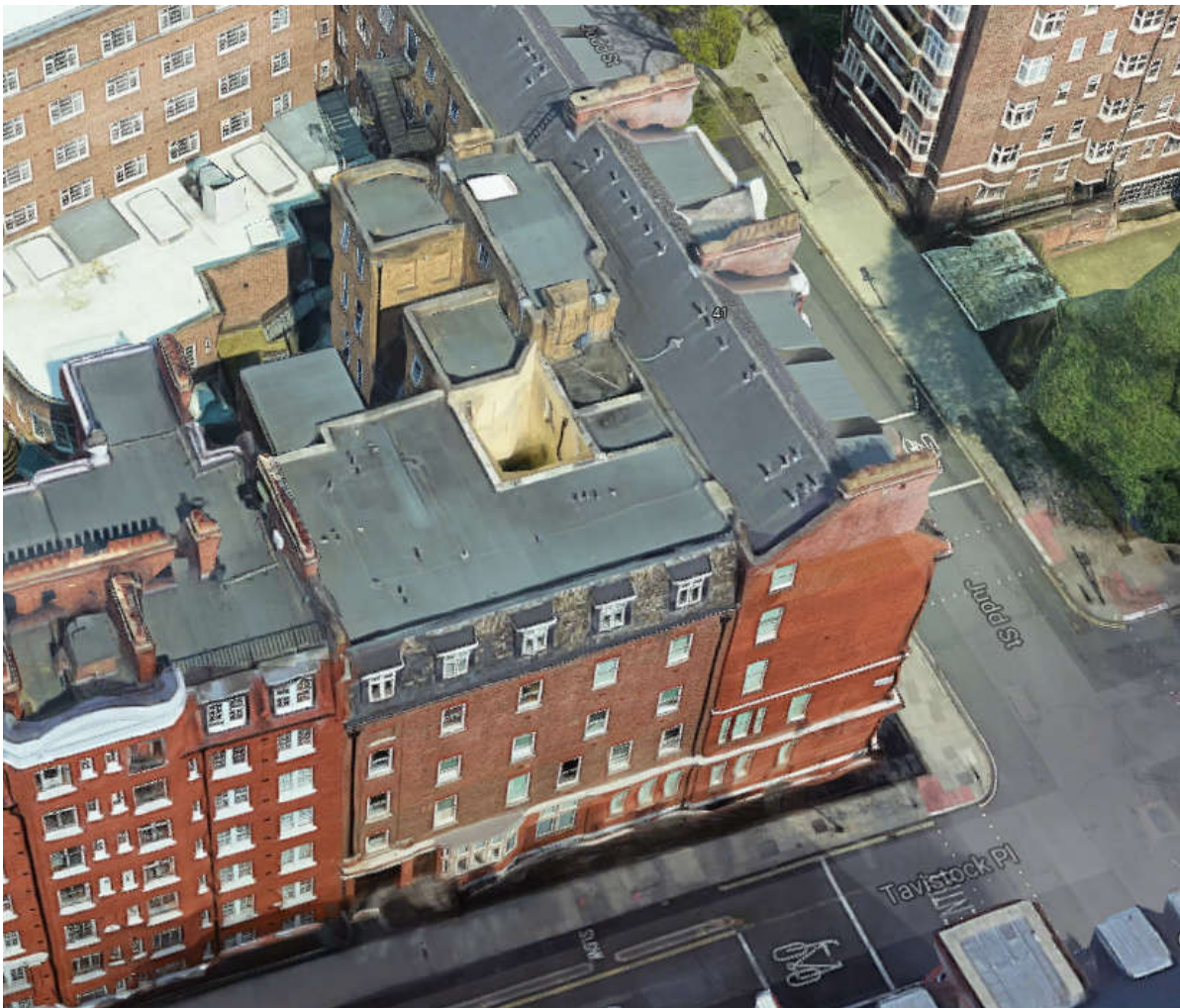
Figure 3 – The majority of the roof on Albany House is flat
