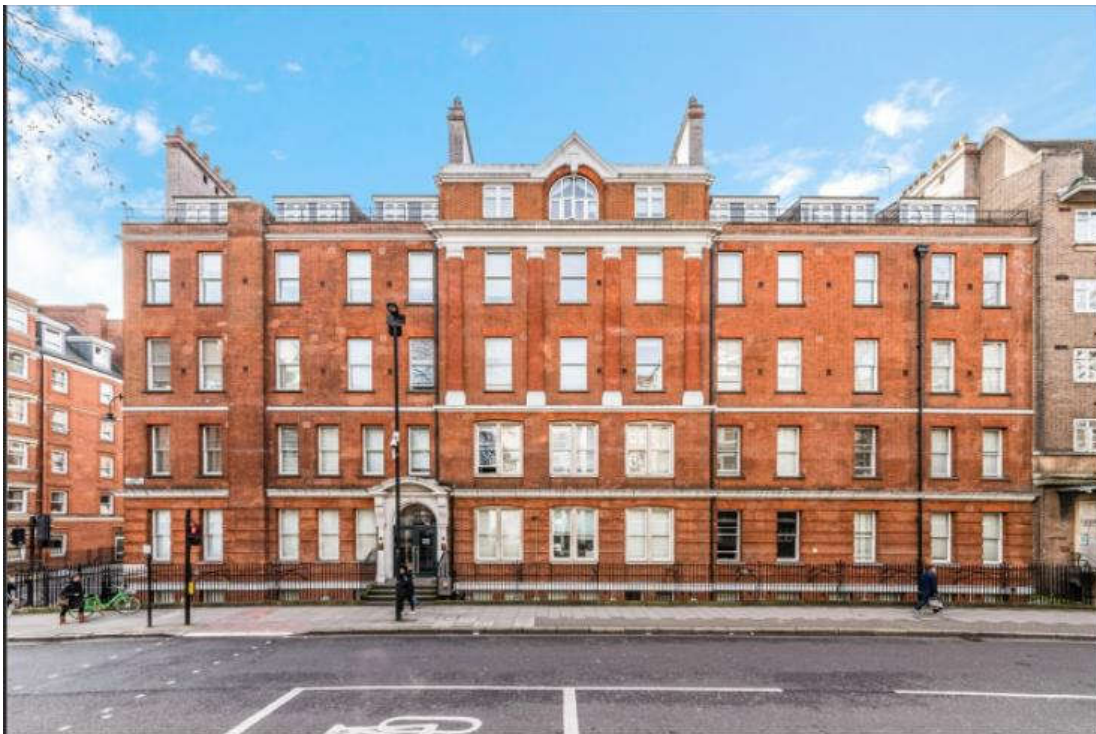
Figure 2 – east elevation of Albany House, which is clearly not designed following the Golden Ratio
