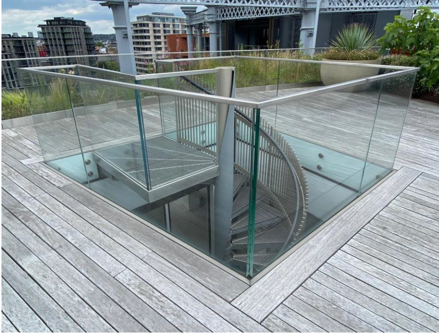
Fig A: Close up of existing balustrade and spiral stair
