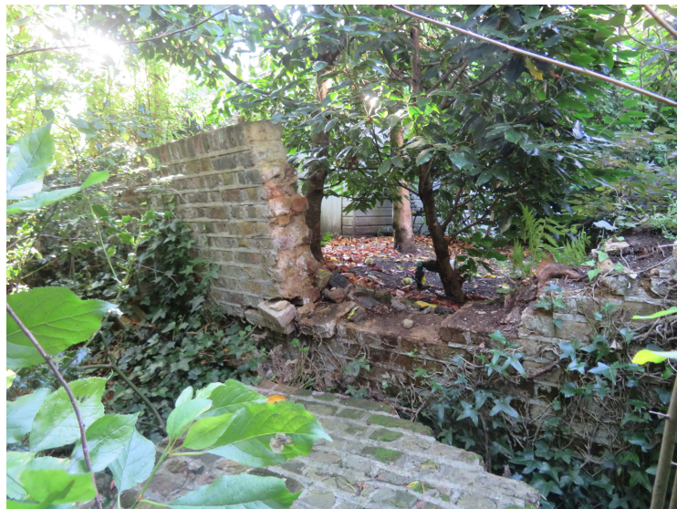
Photograph 1: Showing collapsed wall
