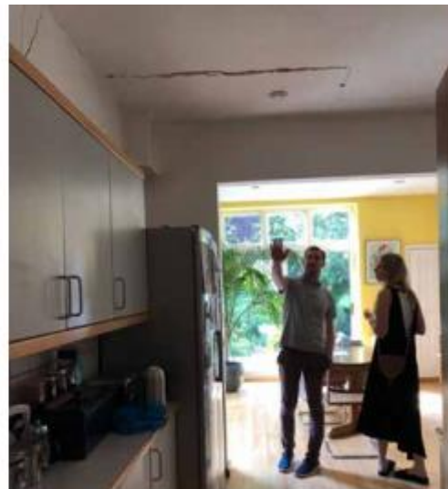
Photo 6 and 7 (above): Views of ceilings and walls of the property showing cracks due to subsidence
