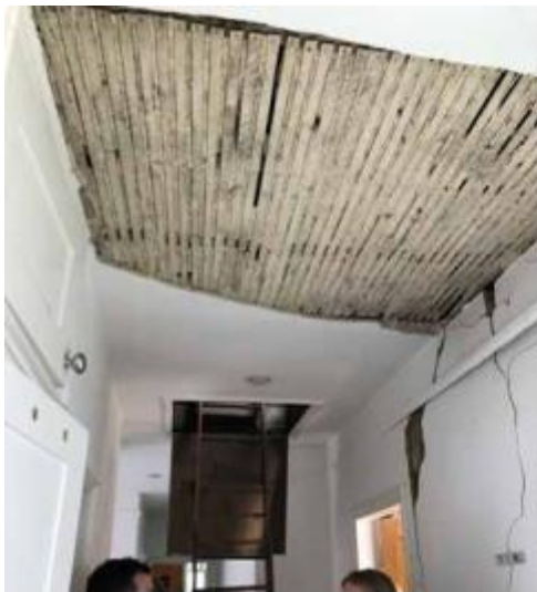
Photo 6 and 7 (above): Views of ceilings and walls of the property showing cracks due to subsidence
