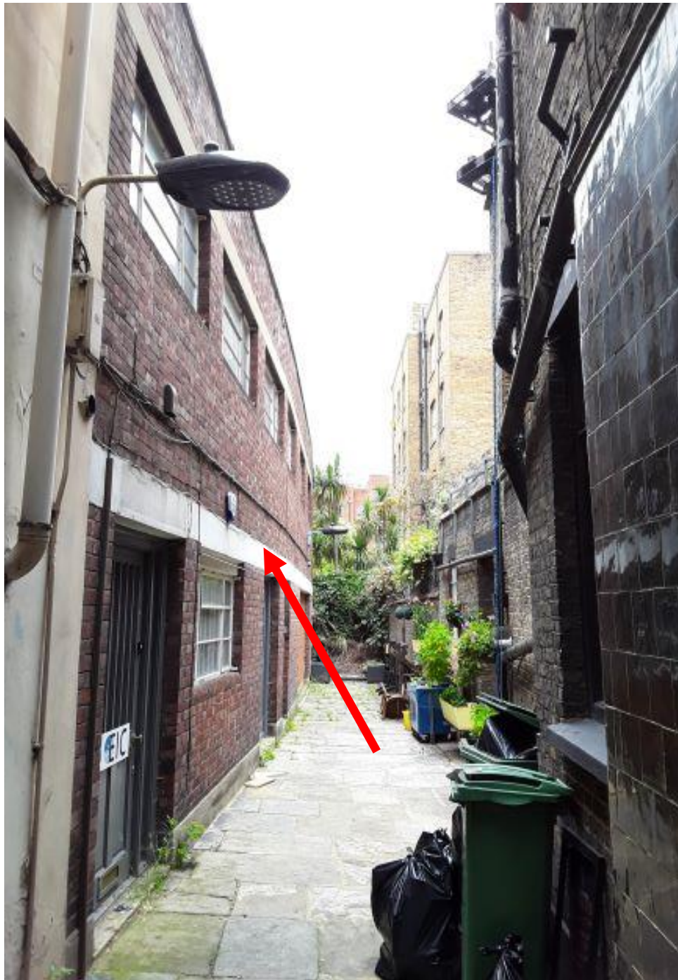
Fig.2 Façade View – July 2021
