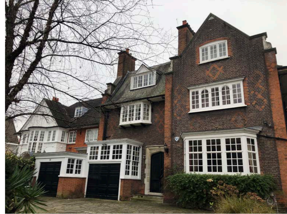
FIGURE.4: PHOTOGRAPH OF THE EXISTING FRONT ELEVATION LOOKING TOWARDS NO.29
