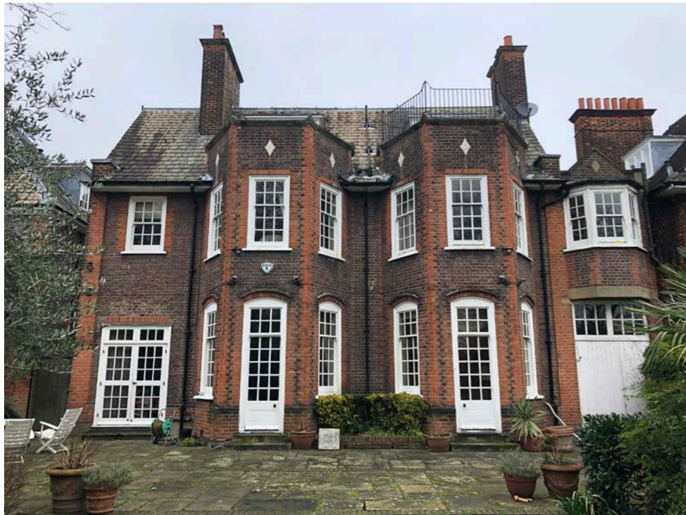
FIGURE.5: PHOTOGRAPH OF THE EXISTING REAR ELEVATION
