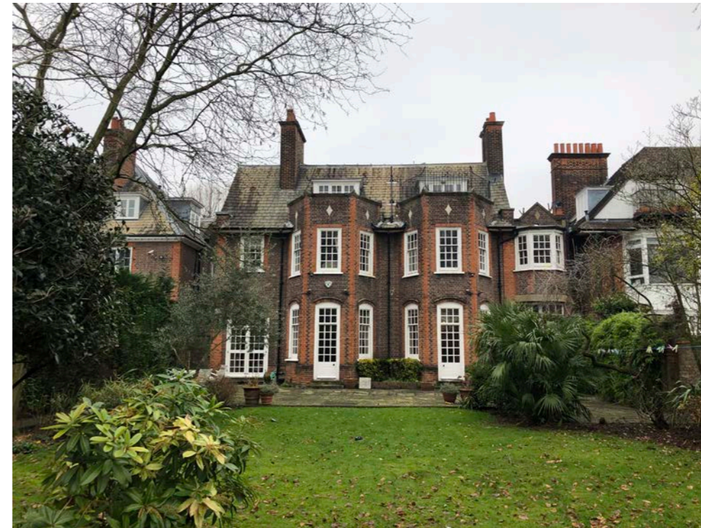
FIGURE.6: PHOTOGRAPH OF THE EXISTING REAR ELEVATION AND GARDEN
