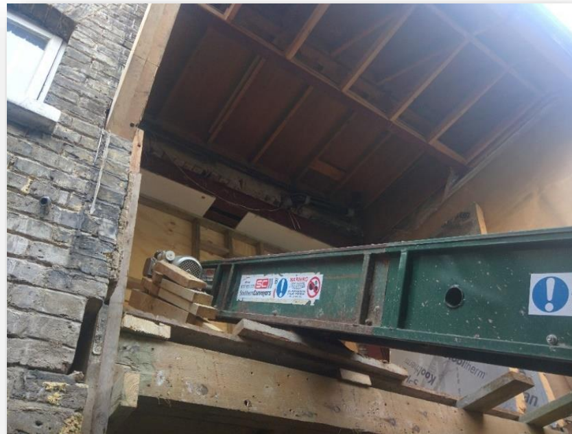
Conveyor to remove arisings
