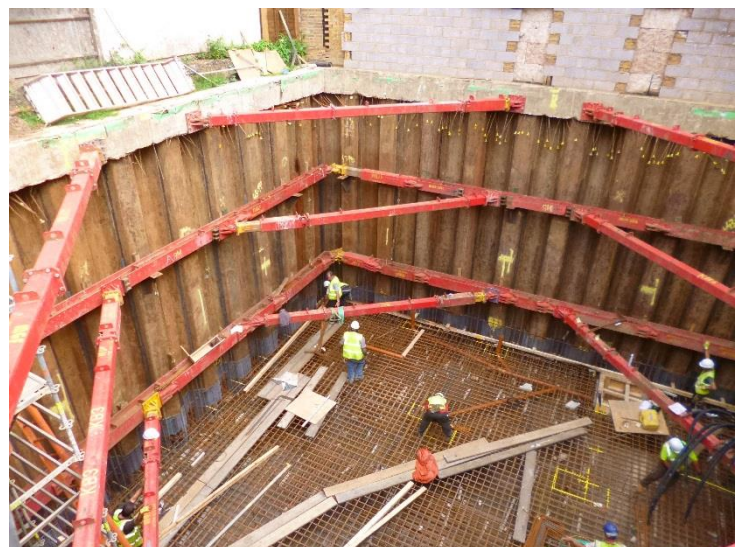
Construction of a Basement within an Interlocking Steel Sheet Pile Wall
