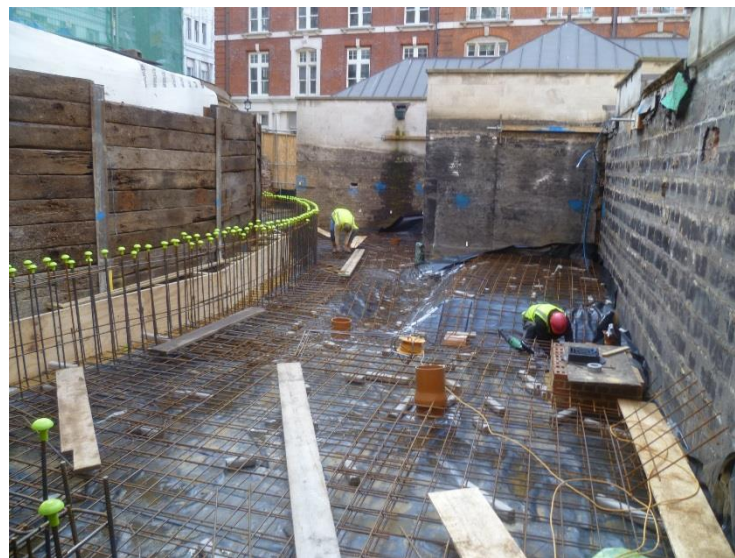
Construction of a Basement within a King-Post Retaining Wall
