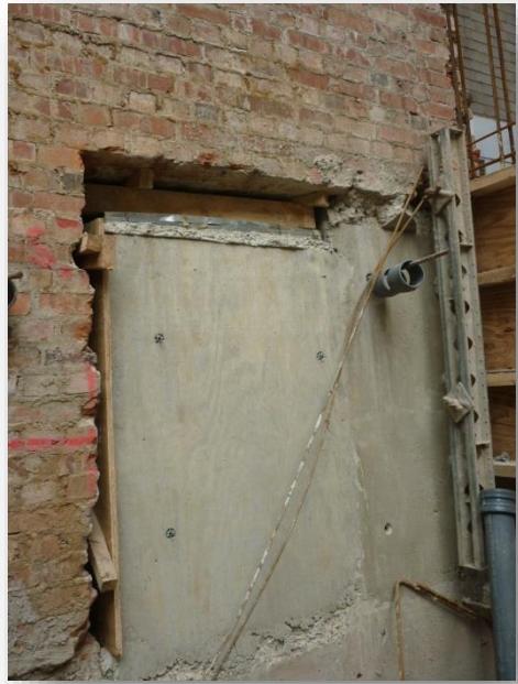
Underpinning To A Masonry Wall
