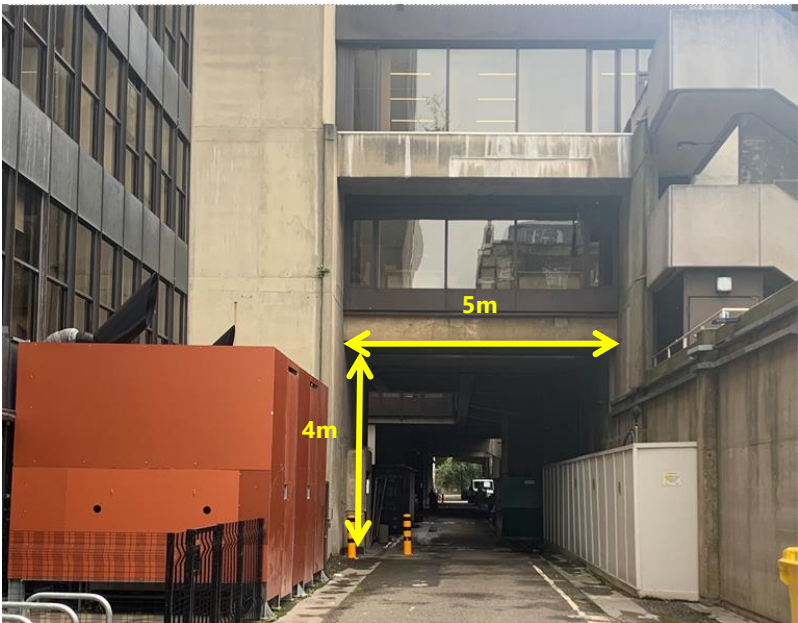
Figure 3—1 Service road tunnel opening (4 by 5 meters)
