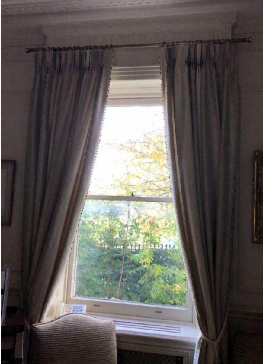
Photo 3: Right-hand side reception room window showing vents for radiator casing
