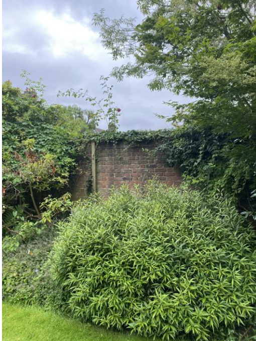
Figure 18: Garden wall, upper terrace, south.
