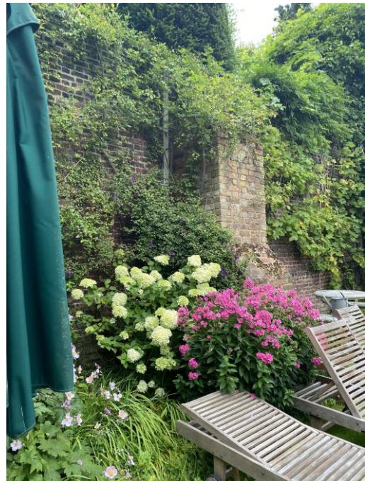
Figure 21: North wall to lower terrace.
