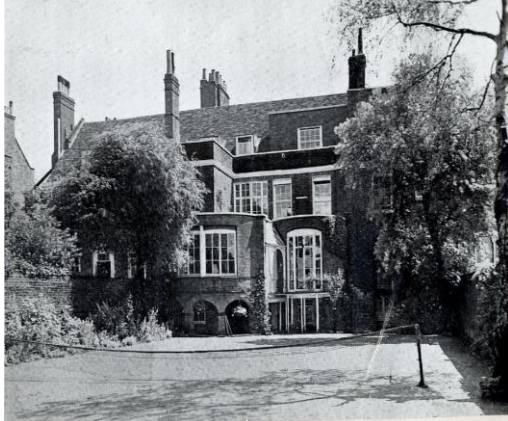
Figure 10: Rear elevation of the original house before reconstruction in the early 1930s.
