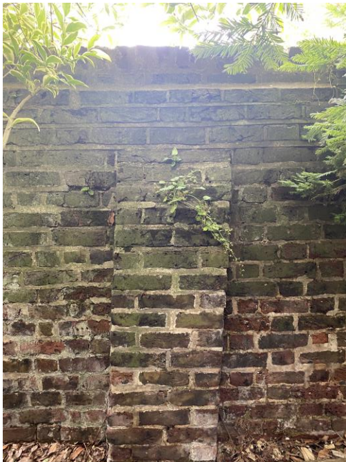
Figure 23: West boundary wall with two brick types.
