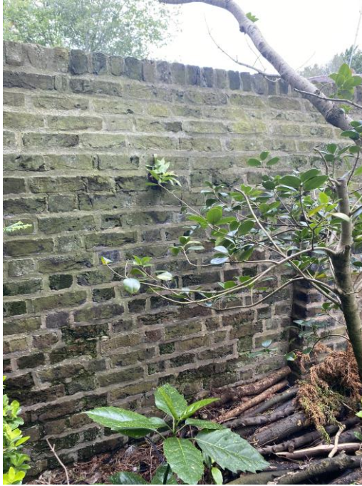
Figure 22: Western boundary wall to the lower terrace.
