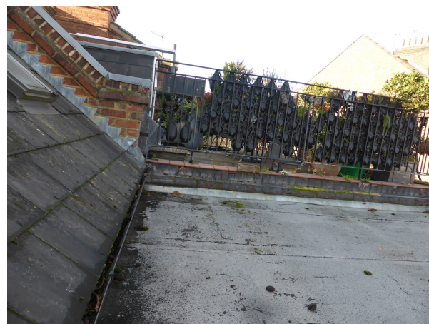
View of adjoining no.31 existing roof terrace
