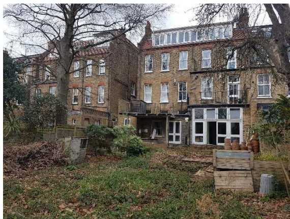
Fig 1: Rear of 65 Greencroft Gardens, London
