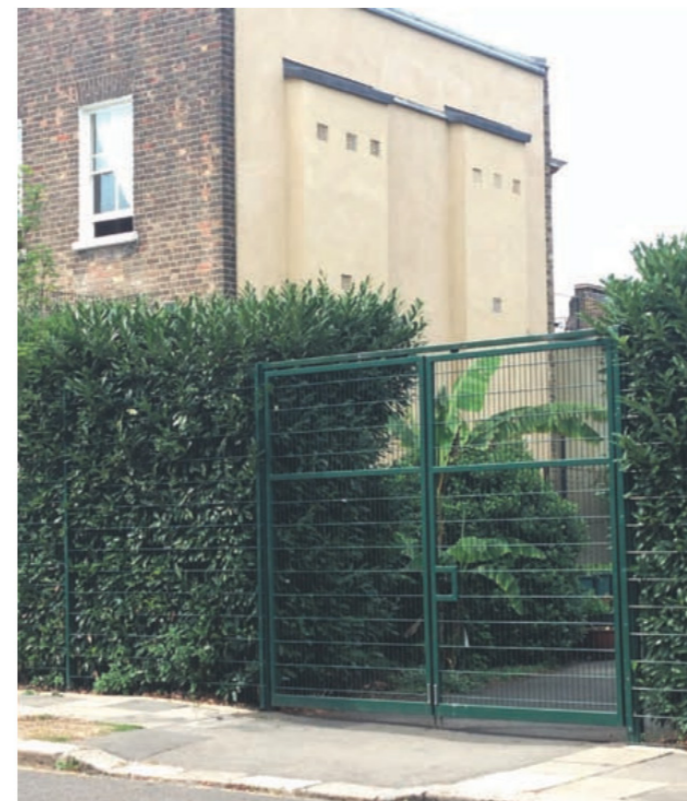
Entrance to site from Marsden Road
