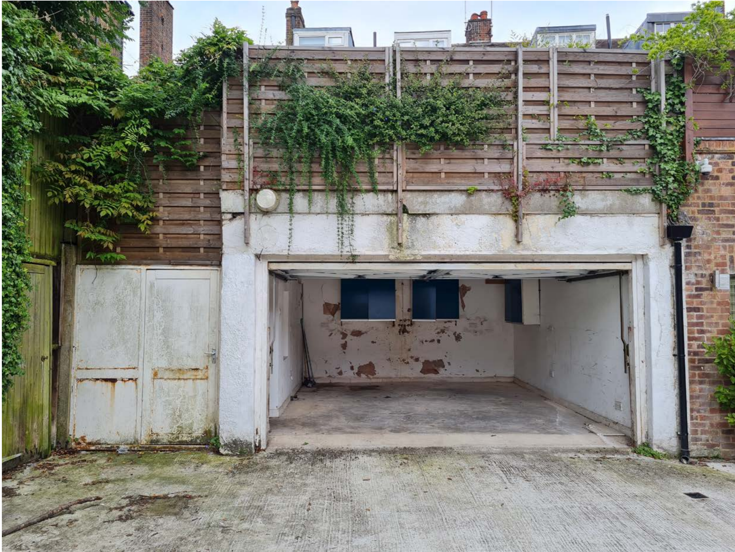
.3 Rear garage elevation from rear dead end access road
