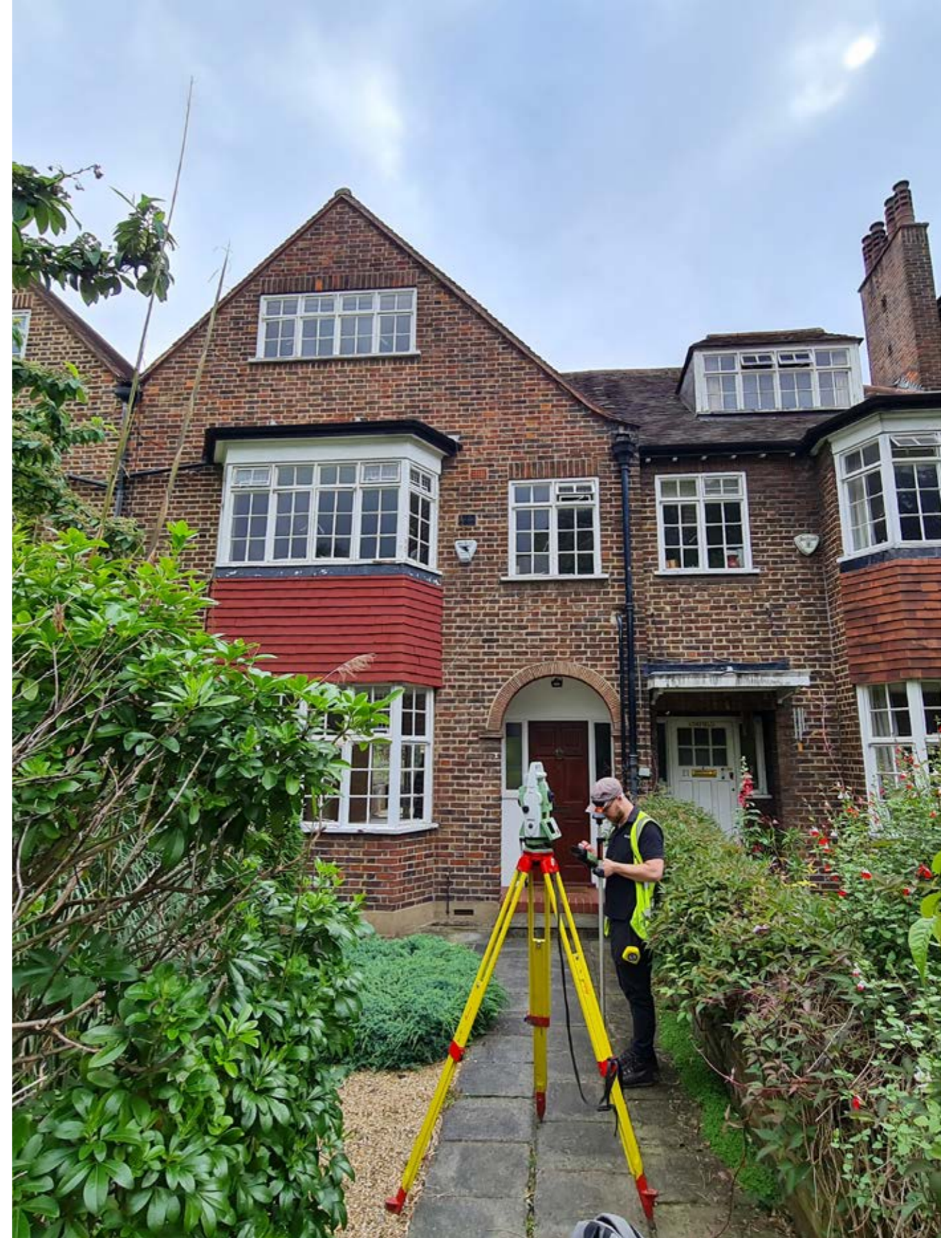
.2 Front elevation from the property entrance pathway 22 Lawn Rd
