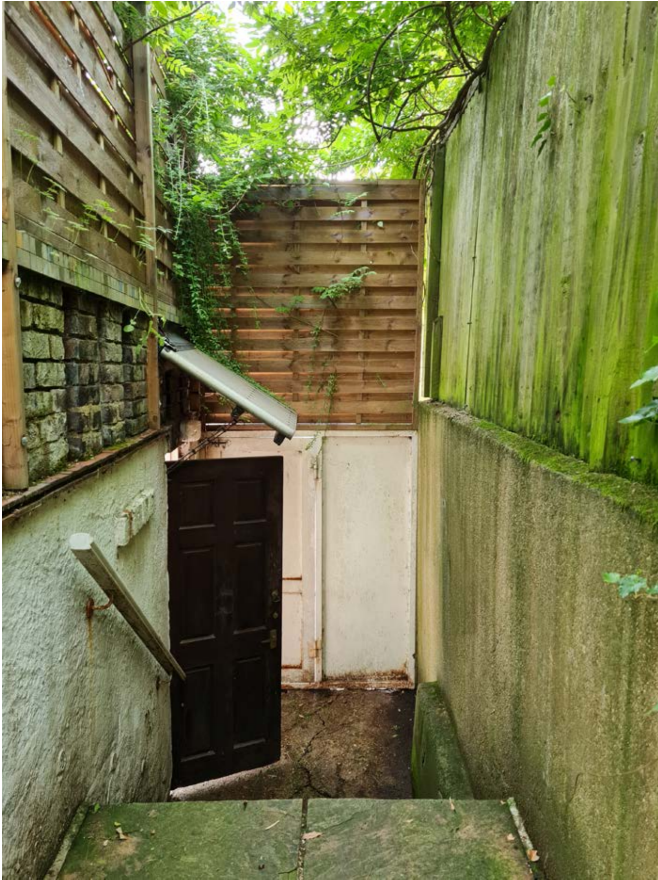
.4 View from external staircase looking down to garage rear access door
