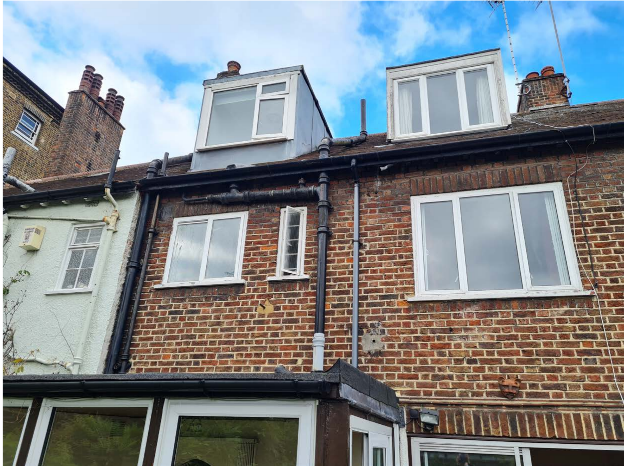
.8 View of the rear elevation first and second floor
