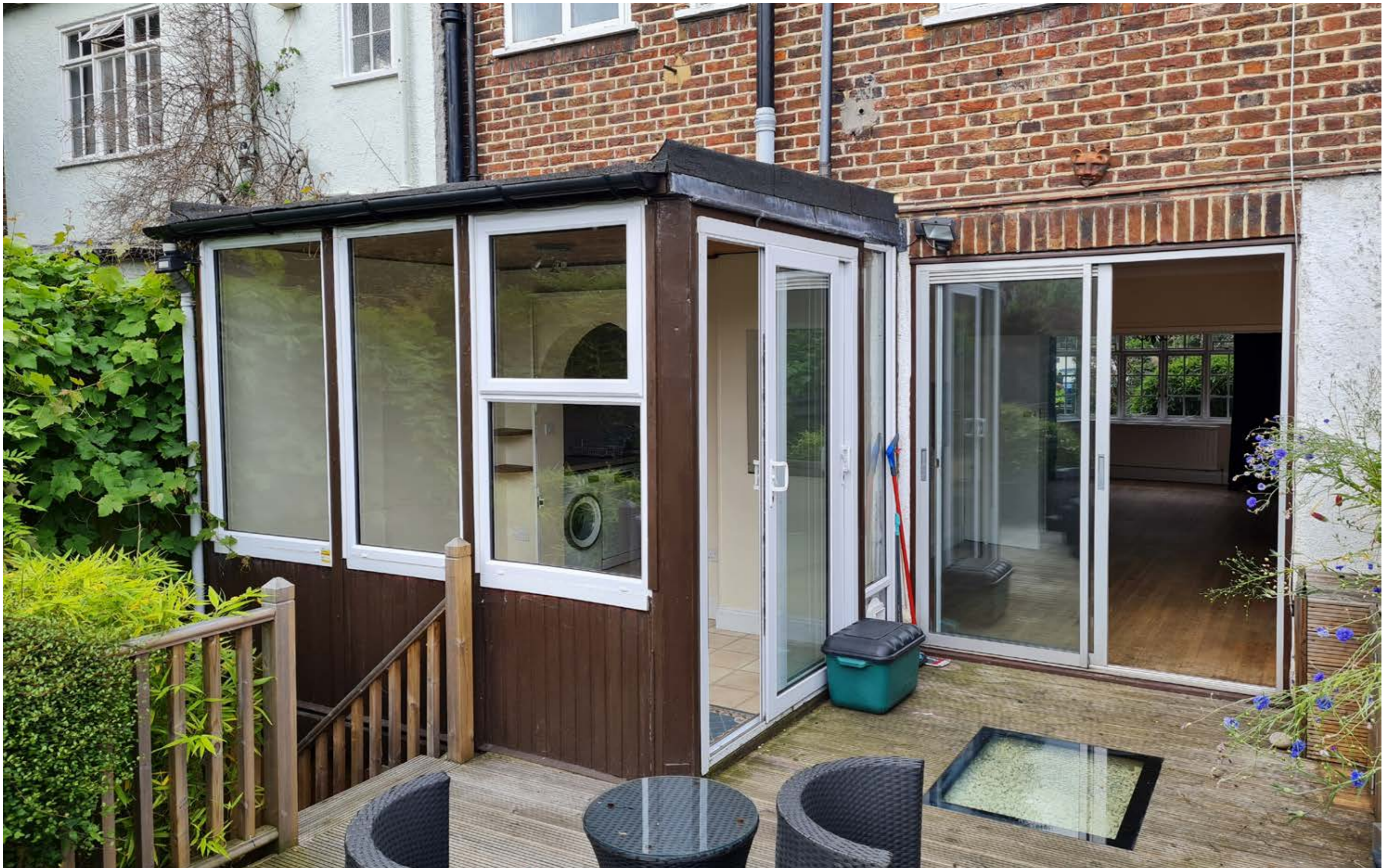
.7 View of the ground floor existing rear extension
