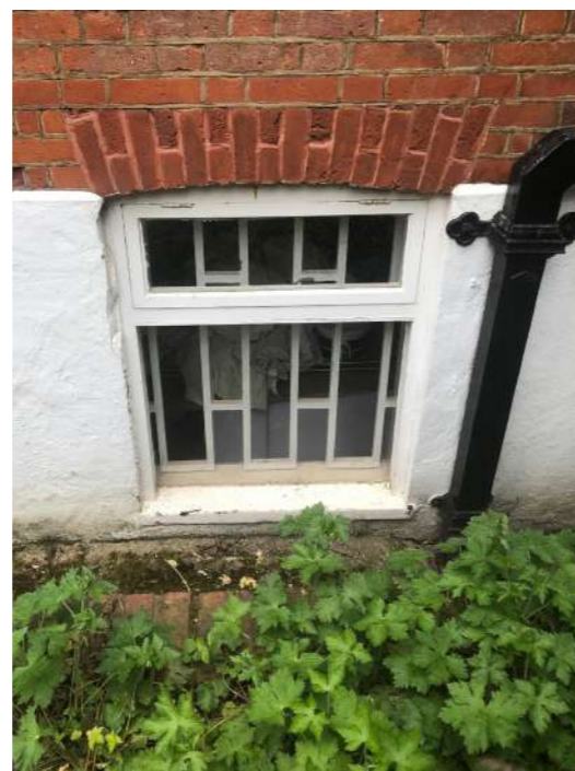
EXISTING WINDOWS IN BASEMENT ROOM
