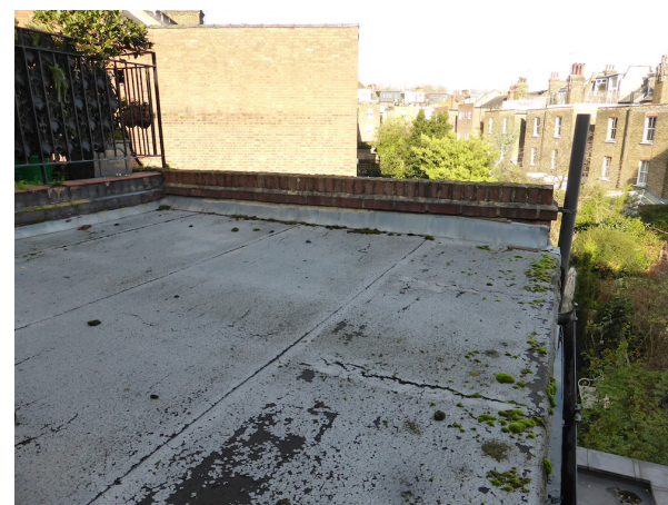
Existing flat roof to no.33
