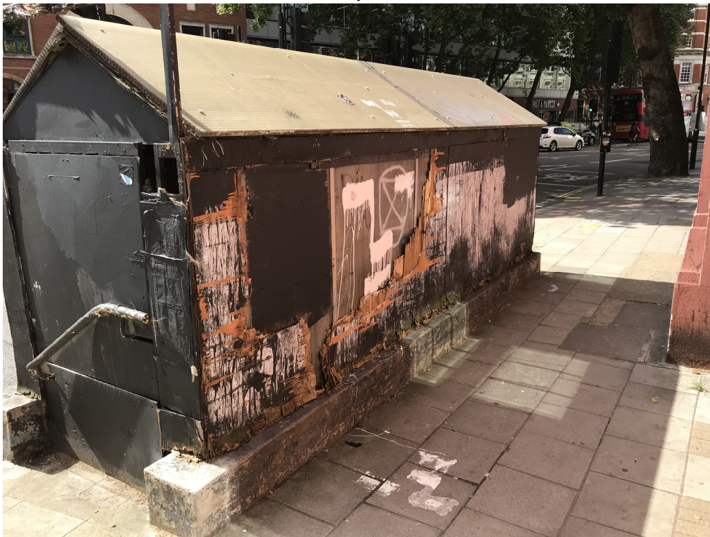
11.2 RHS of Roseberry Avenue Access Point
