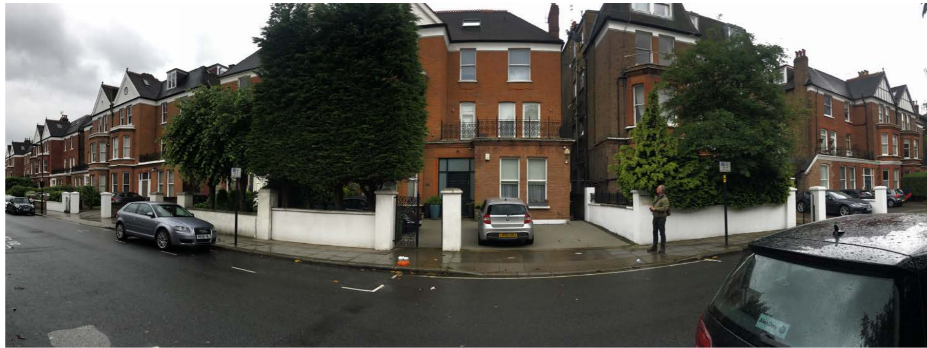
↑ Panoramic view of No.111 Canfield Gardens and its surrounding context
