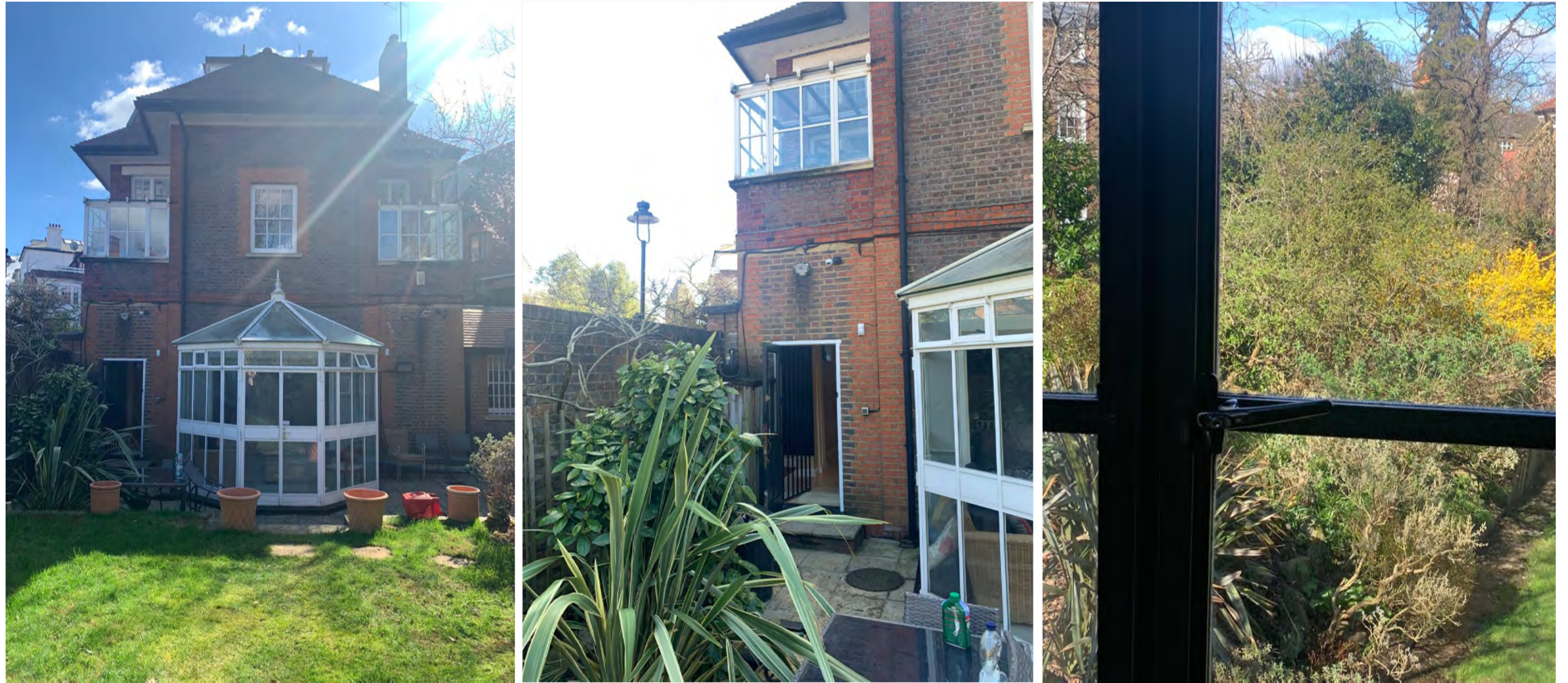
Figures 12 and 13: First Floor Balcony Figure 14: Window detail
