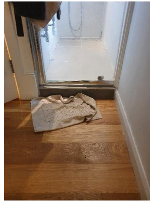
1b. View from the bedroom, no threshold between bedroom and shower room. Platform and glazed door frame require stepping over in order to enter the shower. Intrusive light entering the bedroom
