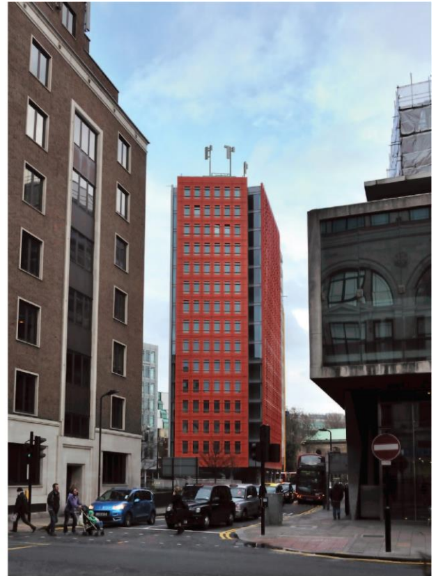
NORTHERN VIEW - ANTENNAS
