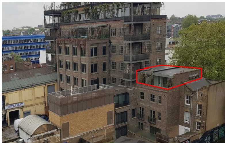
Figure1: Image showing the existing relationship of the balconies at Flat 5 and No. 10 Belmont Street (existing roof and third floor edged in red). Note the existing close relationship between existing balconies, roof terraces and habitable windows. Also note the prevalence of balcony railings and privacy screens and the variation in building design and materials finishes in the locality.
